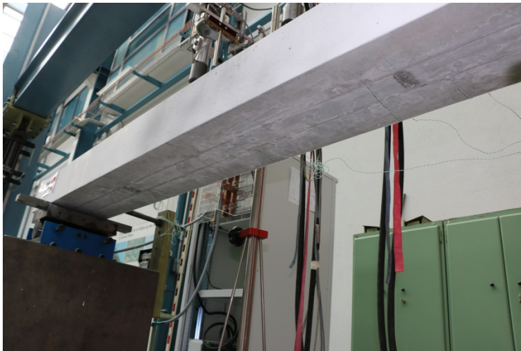
Two strips of SMA embedded on bottom side of a concrete beam for strengthening application (near surface mounted reinforcement).
